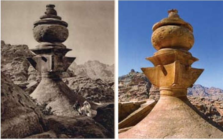
Photographs of the hewn finial on al-Deir (the monastery) shot in 1928 (left) and 2005, show little natural deterioration in the sandstone over the past 75 years.
